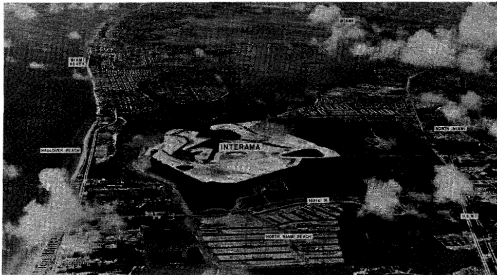
The Site Today, After Clearing and Filling
