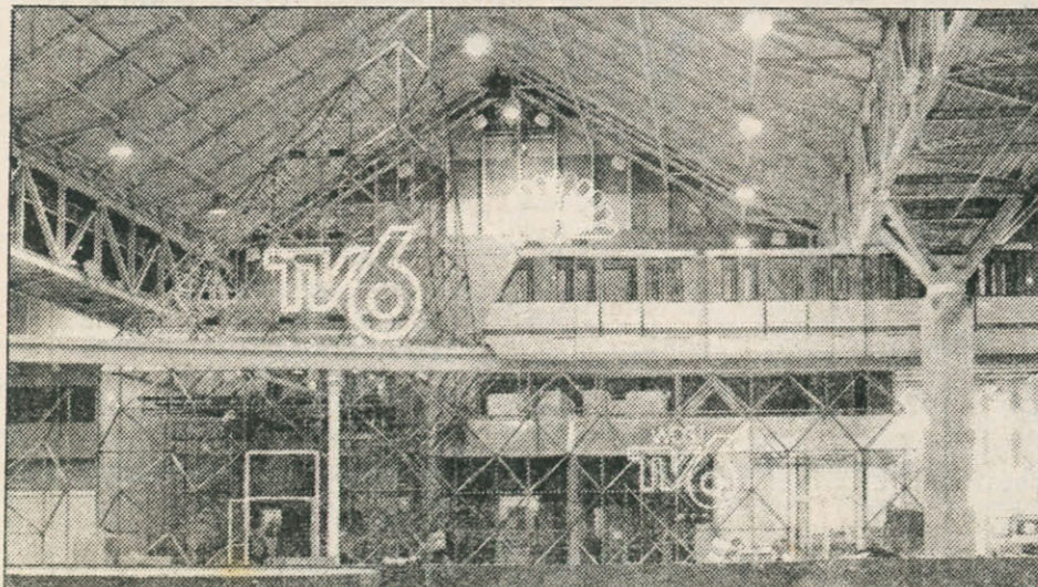
The TV6 Telecommunications Center at the fair
