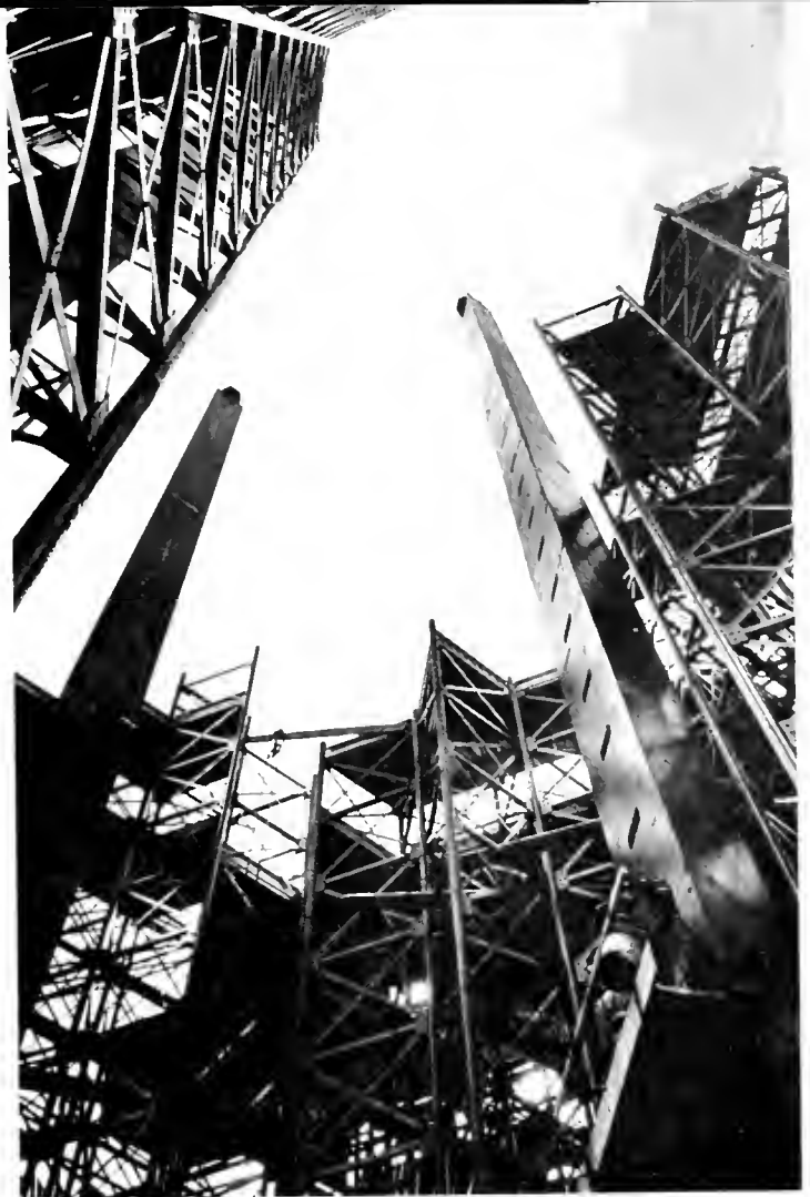
Above: steel-framed prism staggered vertically to 80-foot high form complex of geometric shapes housing Electric Power and Light exhibit. Below: Simmons Company exhibit utilizes this structural steel frame designed as an "oasis of tranquility" symbolic of the trade name "Beautyrest."
