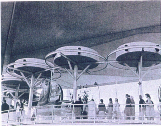
FESTIVAL OF GAS Pavilion is uniquely lighted by 170 1000-watt R-80 color-corrected mercury vapor lamps, mounted on top of the restaurant, fun house, and cupolas in the Carousel area, directing their light to the soaring roof five stories above the ground.
