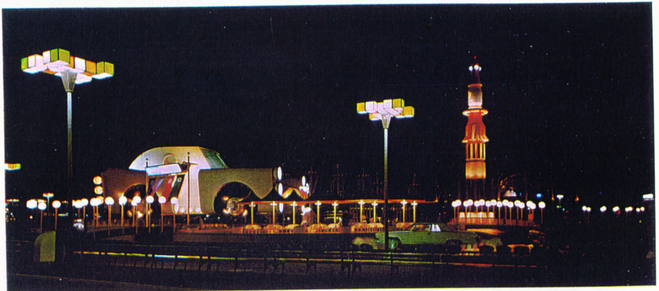
FESTIVAL OF GAS Pavilion is uniquely lighted by 170 1000-watt R-80 color-corrected mercury vapor lamps, mounted on top of the restaurant, fun house, and cupolas in the Carousel area, directing their light to the soaring roof five stories above the ground.
