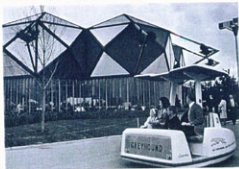
Minnesota building's striking appearance is partly due to sandwich panels consisting of rigid vinyl, made by Monsanto's Building Products Department, with a foamed plastic core.
