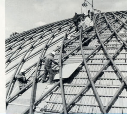
A lamella steel pipe dome crowns the General Electric Company Pavilion
