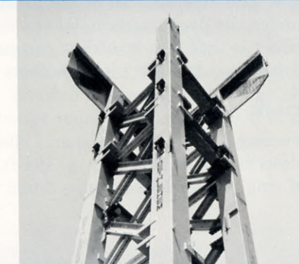
Lofty steel towers support eight giant trusses for the United States Pavilion
