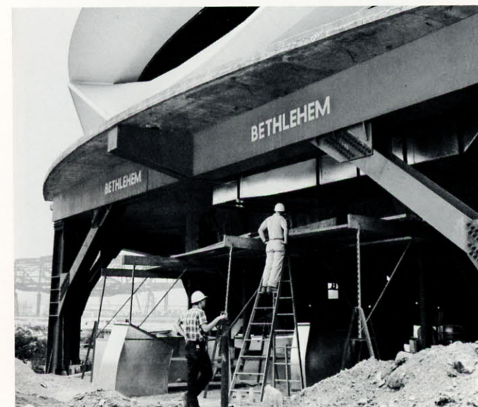
Massive steel bents, all-welded except for the field-bolted knee braces, frame the entrance-exit arches.
