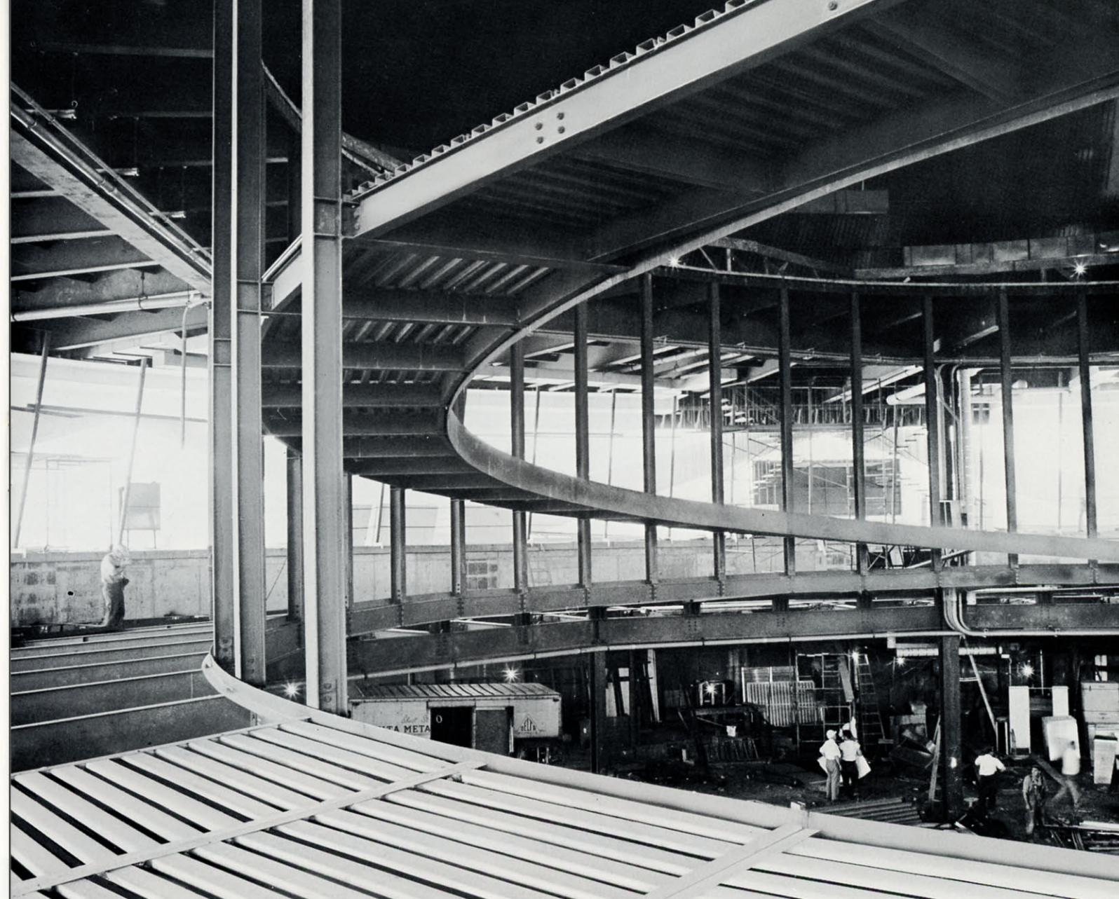
View from the second level. Steel decking for one of the stages is in the foreground. Framing for the circular ramp is cantilevered from vertical hangers. The ramp will bring visitors down to ground floor exhibits from which they proceed to the exits.
