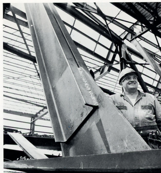
The heavy diagonal members shown here help transmit the "kick" from the long U-frames.
