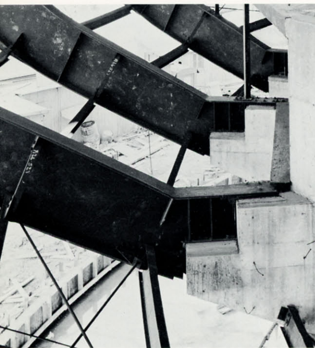
Note the extremely light structure of the footings and lower portions of the ribs.
