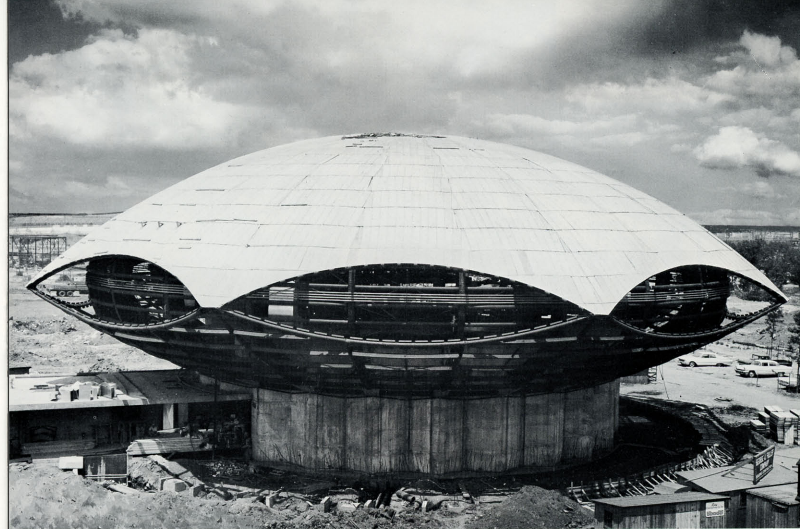
Note how the addition of outriggers and miscellaneous steelwork transformed the basic spheroidal shape into that of an umbrella mirrored by a similar shape below.
