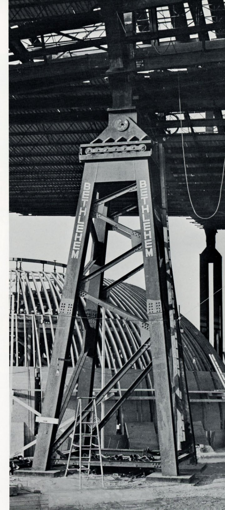
One of the two front, trussed pylons. It is the only support equipped with rollers to permit slight movement, horizontally on the "wing's" longitudinal axis.
