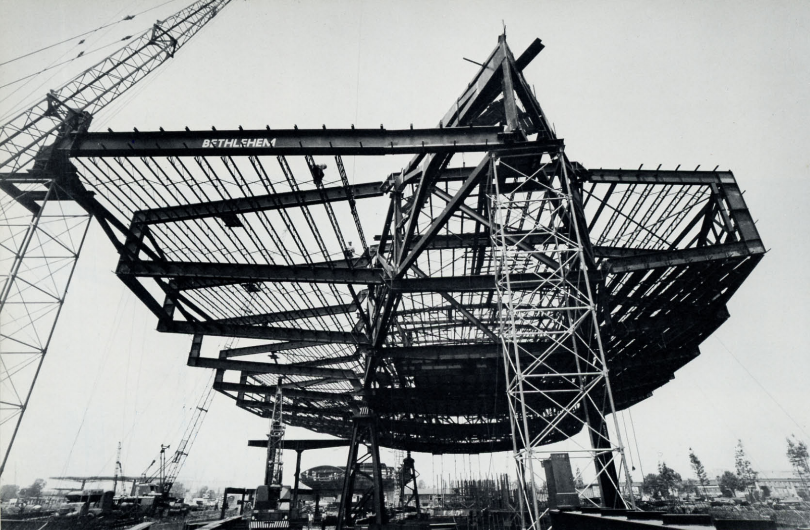
The transverse frames at the extreme ends were erected after all U-frames were in place. The completed structure gives no outward hint of the pointed effect so evident in this picture.
