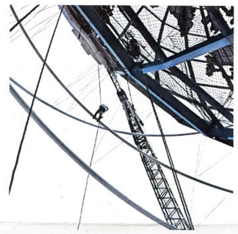
plates. All connections for the Southern Hemisphere are field welded. Three stylized orbit rings that circle Unisphere are anchored by thin stainless steel aircraft cable, barely visible from the ground.
