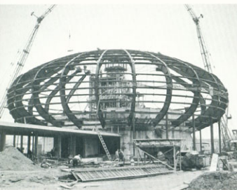
Next step was to erect the upper halves of the ribs (welded splices), and install purlins. Meanwhile, the tension ring was positioned on falsework. When all cables were tensioned, the basic structure was complete.
