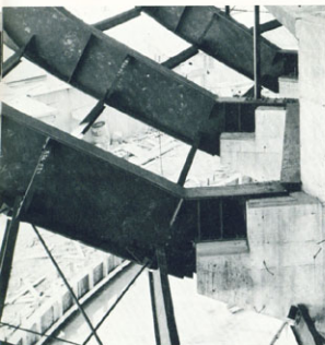
Note the extremely light structure of the footings and lower portions of the ribs.
