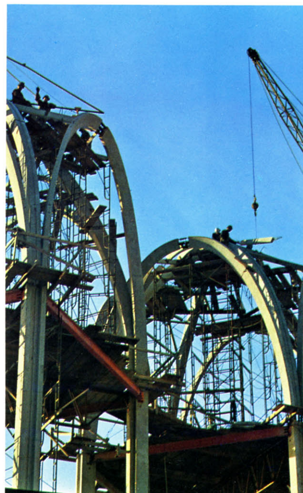
The arches at the Science Exhibit are fitted in place.
