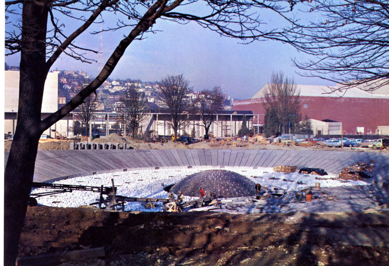
February, 1962: Construction crews install lighting fixtures in the huge International Fountain.
