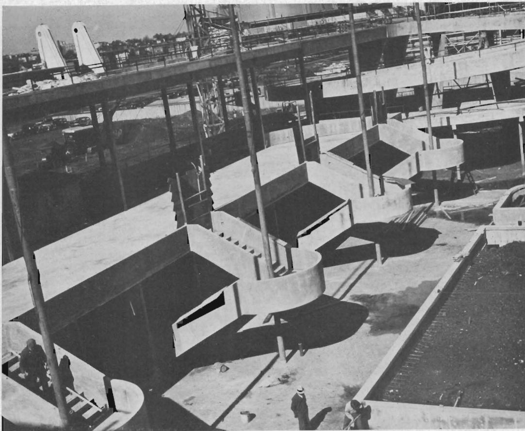
Entrance to loading platform of "roof ride" is by means of cantilevered concrete stairs.
