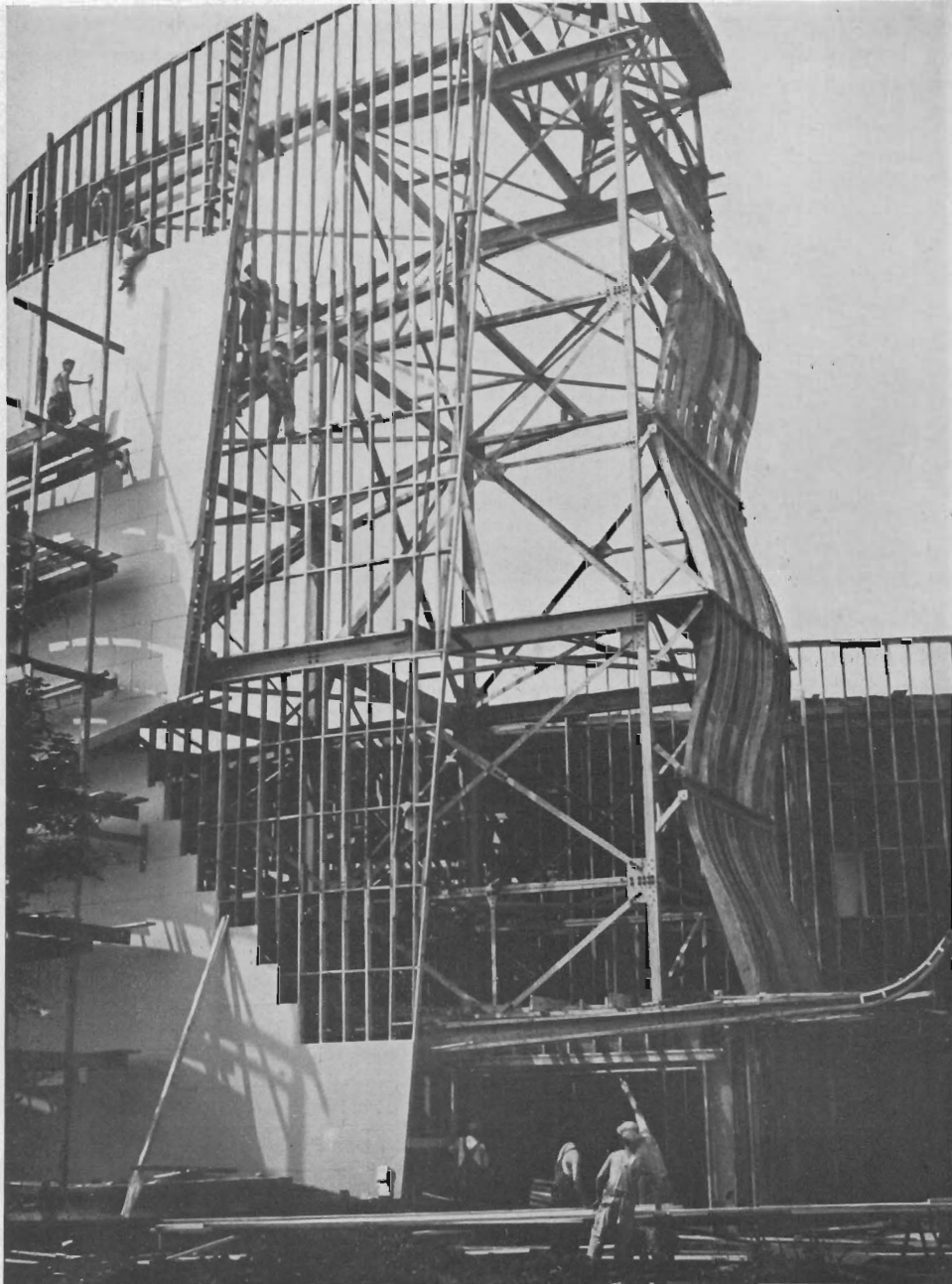
Steel framing, timber studs, and plasterboard. Main entrance, Hall of Pharmacy.
