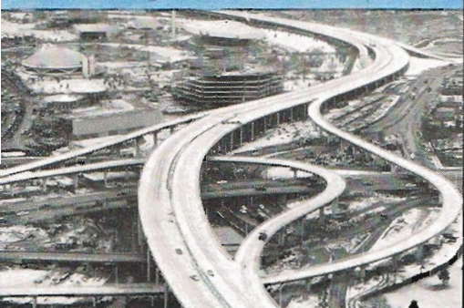
Van Wyck Expressway Extension
